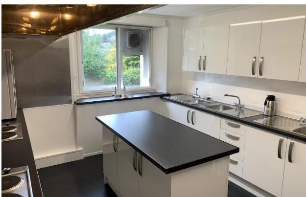
Refurbishment of the kitchen, dining room and lounges at Pitlochry YH.
